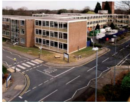
B424 Prior to demolition
