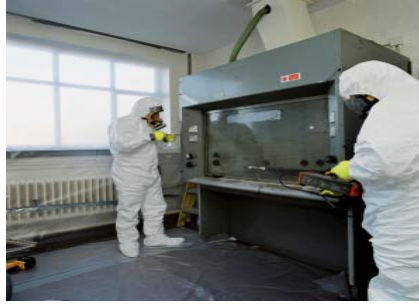
Post Operational Clean Out.
