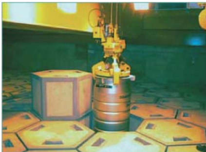
Placement of cemented waste in the TRS
