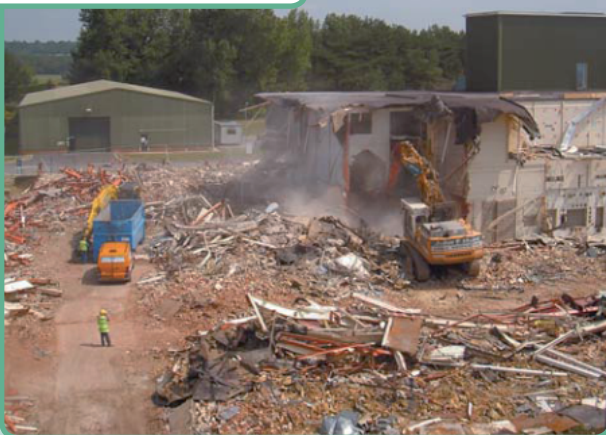
Progress in the Demolition of Building A59
