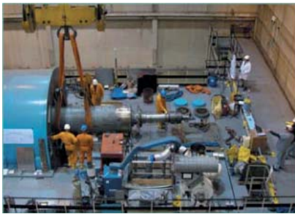
Turbine rotor removal at SGHWR
