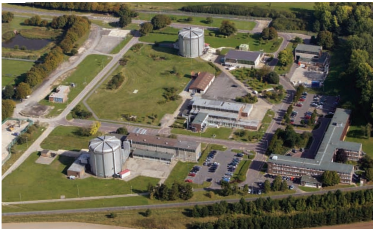
The 'reactor area' of Harwell. PLUTO and DIDO are clearly visible, LIDO has been removed, as have many auxiliary plant buildings
