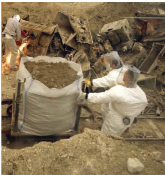
Excavation of the beryllium disposal pits
