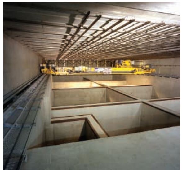
The intermediate-level waste vault store at Harwell
