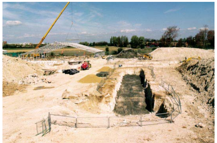
Beryllium disposal pit after removal of waste showing clay liner
