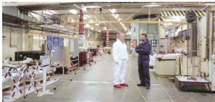
Active handling building following decommissioning of shielded cells
