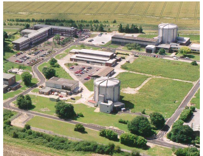
Harwell 'reactor' site after decommissioning
