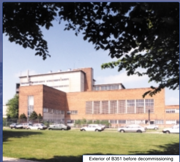
Exterior of B351 before decommissioning
