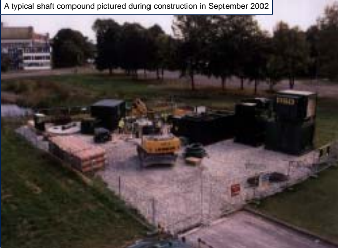
A typical shaft compound pictured during construction in September 2002
