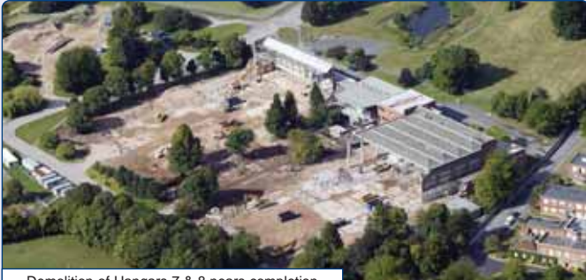
Demolition of Hangars 7 & 8 nears completion
