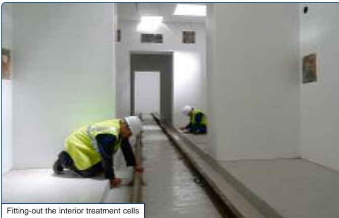
Fitting-out the interior treatment cells
