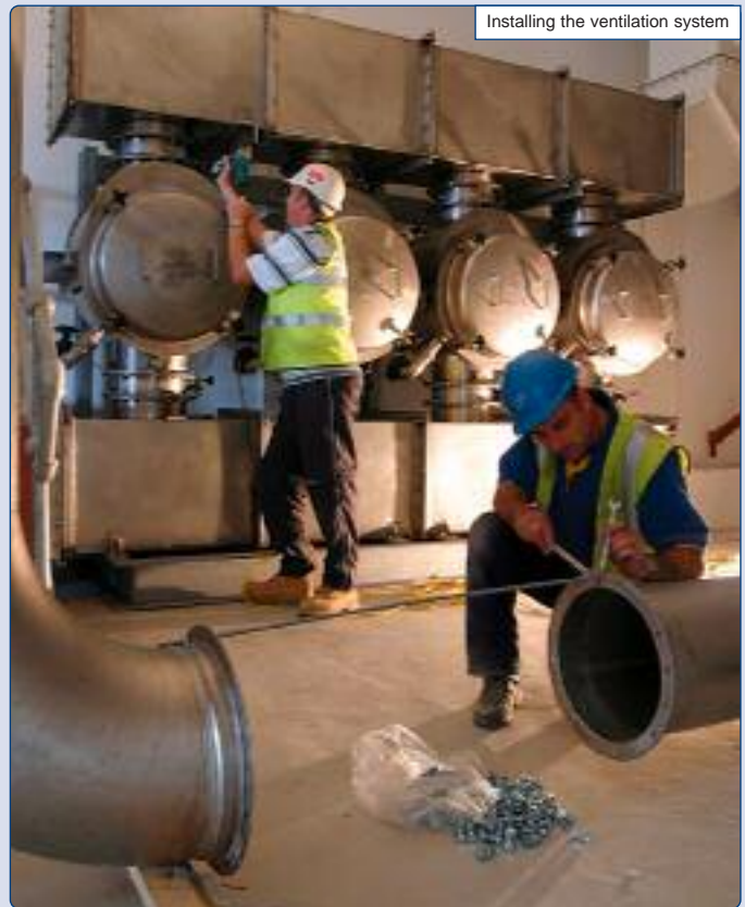
Installing the ventilation system
